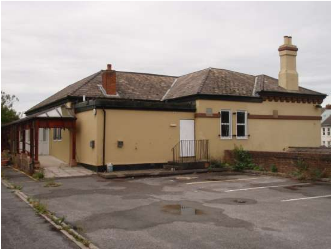
Plate 8. Rear view of Site (looking West)
