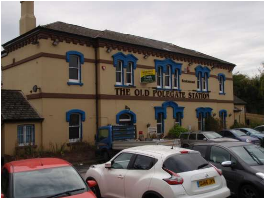
Plate 4. View of Station (looking SW)
