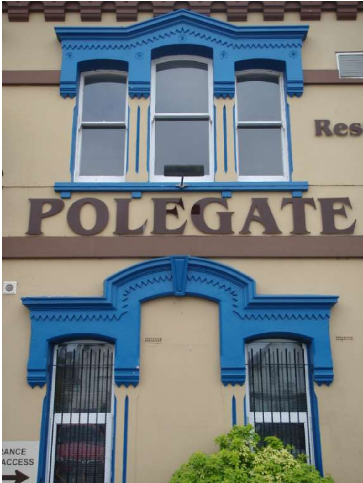
Plate 7. Detail of Old Polegate Station (looking South)
