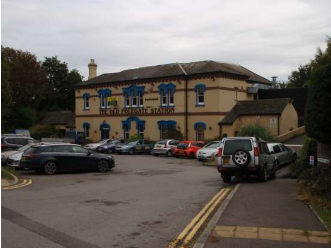
Plate 5. View of Station (looking SE)
