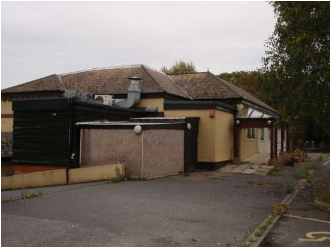
Plate 9. Rear view of Site (looking East)
